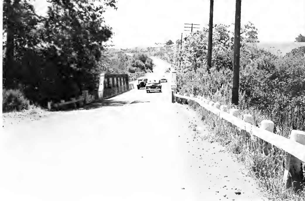
Old narrow bridge across Dos Pueblos Creek was replaced by modern structure
